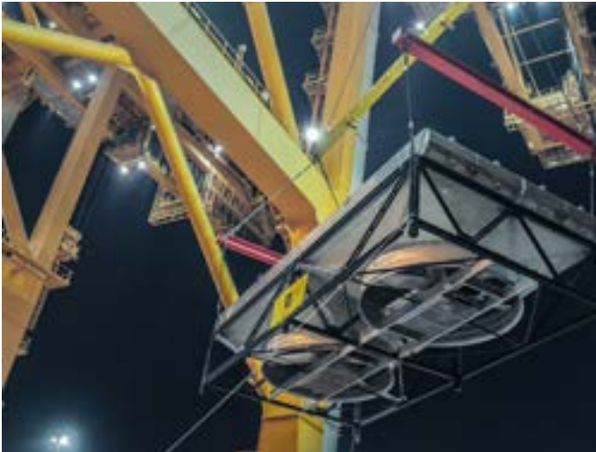
8 Heat exchangers shipped from Jebel Ali to West Africa using shore Gantry crane.
